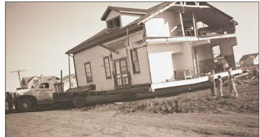
Right: Moving the Spirit River Immigration Hall. The building was too large to move in one piece, so it was split down the middle, allowing you to see the interior of the building as well. (SPRA 676.03.03.09.143)
