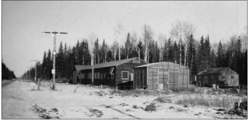
The long low log building above is the Royal Canadian Corps of Signals Repeater Station at Little Smoky during the second World War. Behind it is the maintenance building, and the weather station. SPRA 294.02
