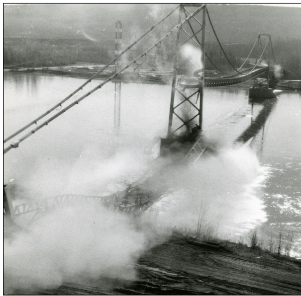
Above: The Collapse of the Taylor Bridge (SPRA 032.08.08.1147 )
