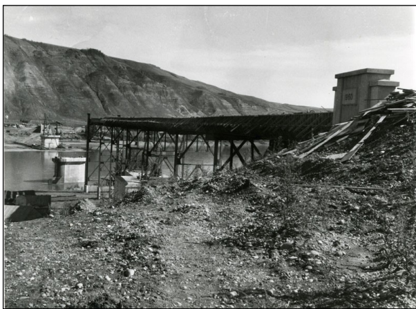
Above: Dunvegan Bridge under construction in the summer of 1960. (SPRA 2000.73.102 )
