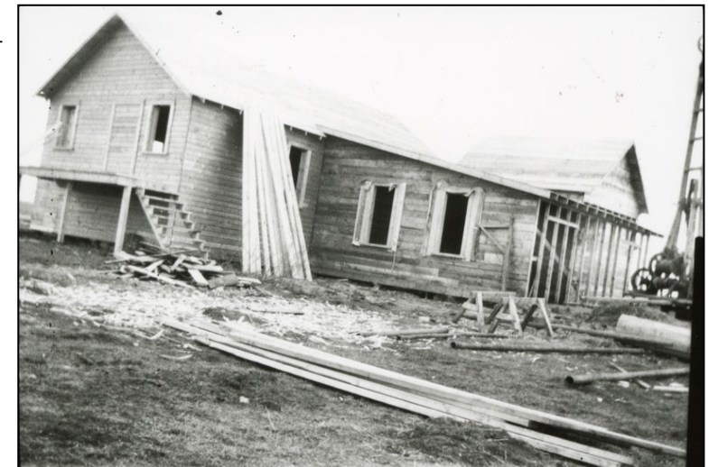
Right: Building the Creamery in Valhalla, ca. 1918 (Fonds 355, 2009.082.49)
